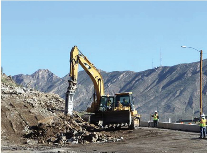
Top: A breaking hammer pummels the side of a mountain along Sun Bowl Drive as part of a widening project that will make the popular north-south corridor safer, especially during special events when traffic demands increase.
