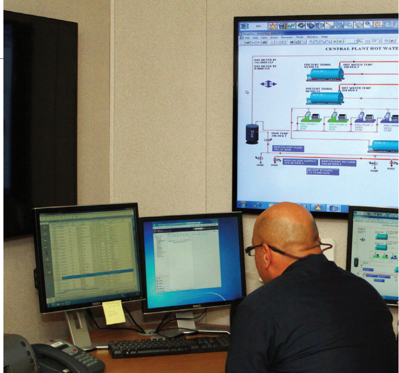
Manuel Arzate, operator I, monitors the central plant hot water system from the Campus Central Control Center. Operators such as Arzate keep track of the temperatures in each building, the operation of the thermal plants, the fire alarm systems and the research support monitoring systems to make sure they are running efficiently.
